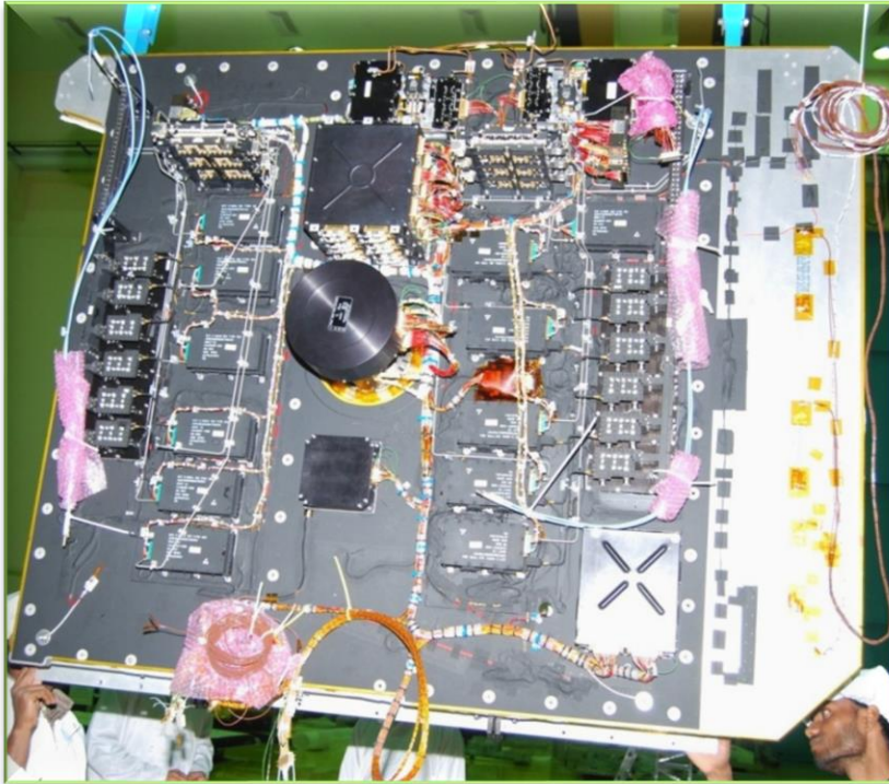
SOUTH PANEL READY FOR ASSEMBLY
